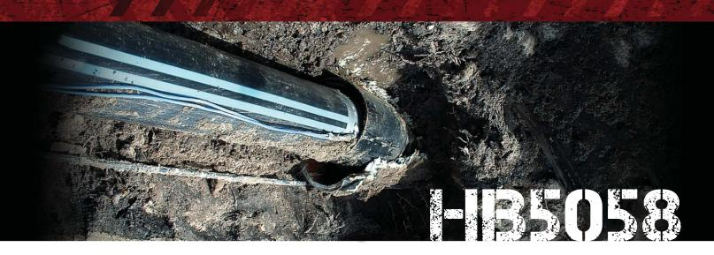
**COMPACT AND EFFICIENT.** The HB5058 gives you up to 50 tons of pulling power in a compact, highly efficient bursting system. It's simple to set up, easy to operate and leaves a small footprint. Its quick replacement jaw inserts, onboard pressure gauges and auto rod grip-and-release make the pipe bursting operation as simple and efficient as it can possibly be.
