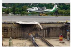
Project: Pipe bridge culvert under military runway Specifications: 26 rams of 24" steel pipe 60m Equipment: 16" and 24" pipe ramming hammers
