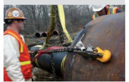
Project: New culvert under Rail track Specifications: 30" & 60" steel casing Equipment: 24" pipe ramming hammer
