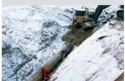
Project: Slick bore – Bannister oil pipeline project Specifications: 360' of 36" steel casing Equipment: 24" pipe ramming hammer
