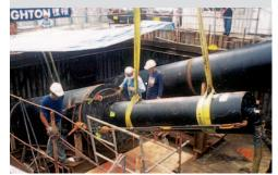
Project: Washover casing installation, HDD assist Specifications: 2 – 54" casings 66' at a 20° angle Equipment: 24" pipe ramming hammer
