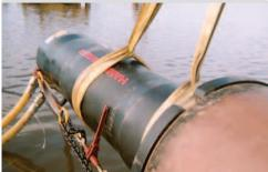
Project: Pullback assist – gas pipeline installation Specifications: 2,800' of 36" casing Equipment: 24" pipe ramming hammer
