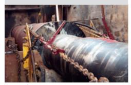
Project: Gas Pipeline (natural gas main) Specifications: 349' of 42" casing Equipment: 24" pipe ramming hammer
