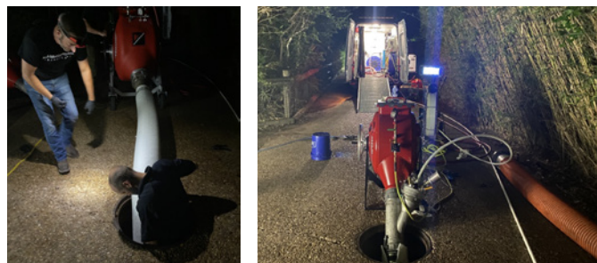
Each 200-foot manhole-to-manhole liner inversion is followed by a transparent calibration tube, which carries the LED head to the other end.
